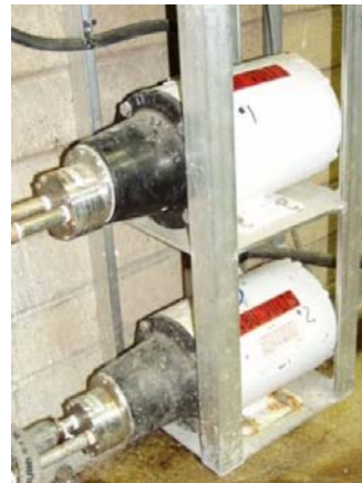
Napa Sanitation District Left: T Tuthill T-series compact installation pumping polymer Right: Tuthill T-series replacing a diaphragm pump for Sodium Bisulfite
