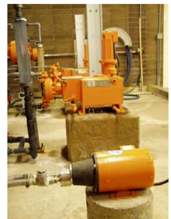
Napa Sanitation District Left: T Tuthill T-series compact installation pumping polymer Right: Tuthill T-series replacing a diaphragm pump for Sodium Bisulfite
